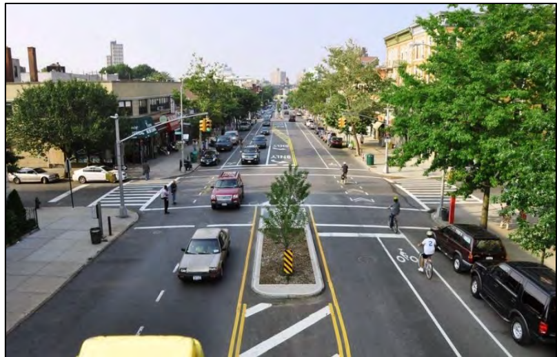
Complete Street example with median, bike lane and left-turn lanes
